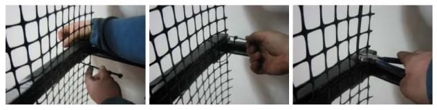
Wrap tie around beam and through mesh ....... Pull tie tight around beam ....... Remove excess with side cutters
