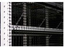
6) If the sides of the grid are unsecured to a post or beam, overlap sections and secure sections together using cable ties. For optimal strength and appearance, RackGuard should be secured at least every 12".
