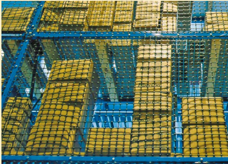
Industrial Netting’s Rack Guard System protects warehouse workers from falling objects.
